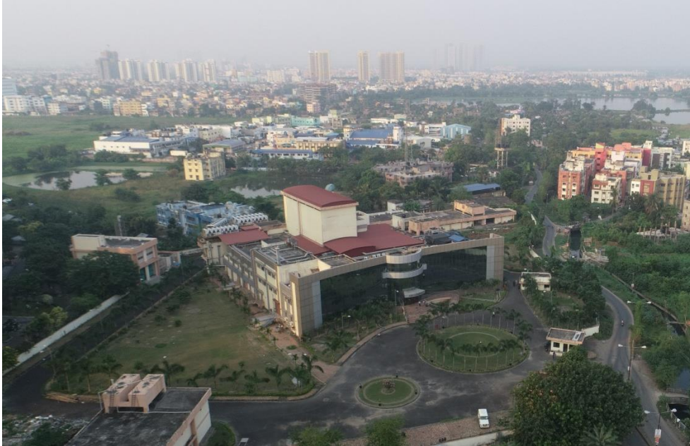
VECC Medical Cyclotron Facility at Chalkgaria, Kolkata
